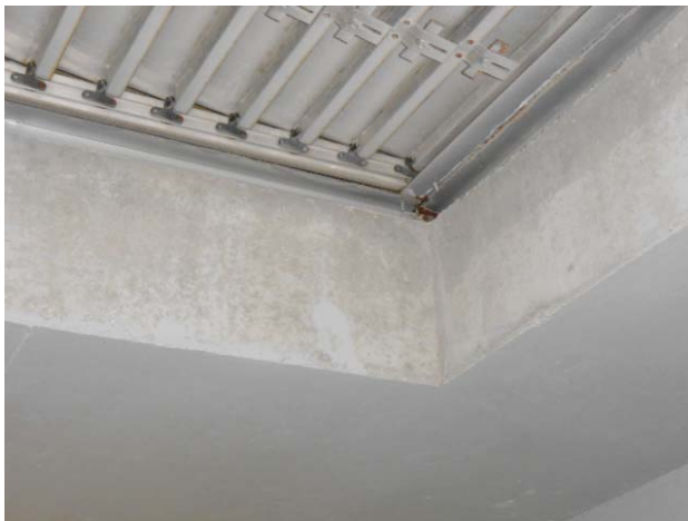
Concrete roof deck
